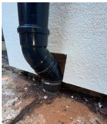
Figure 10 a), b) & c) Various locations of soil vent pipes junctions resulting in thermal bridges
