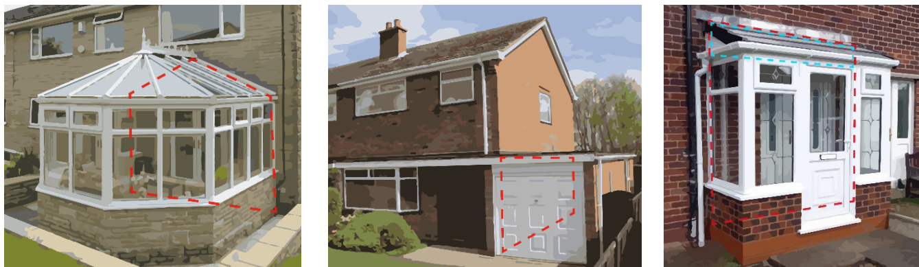
Figure 8 Examples showing the internal heat loss walls in the red and blue dotted area requiring insulating
