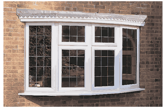
Figure 11 Example of a typical cantilevered bay window
